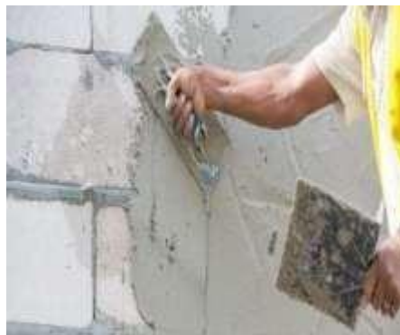
Fig 3: Applying of base coat of plastering for brick masonry
