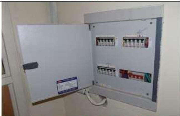
Miniature Circuit Breaker's (MCB's).
