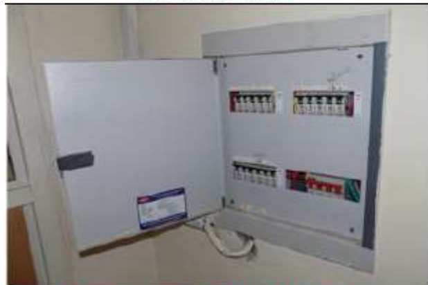
Miniature Circuit Breaker's (MCB's).
