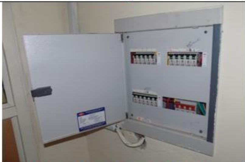
Miniature Circuit Breaker's (MCB's).
