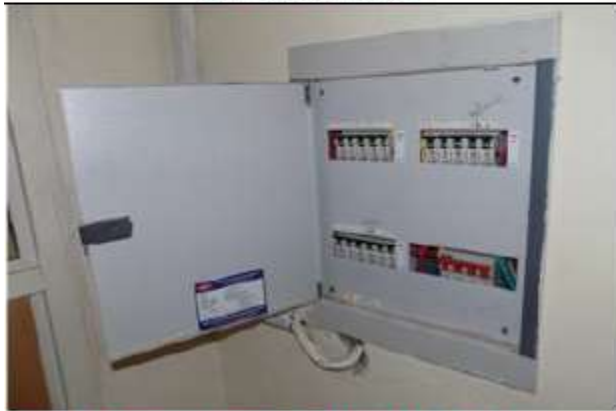
Miniature Circuit Breaker's (MCB's).
