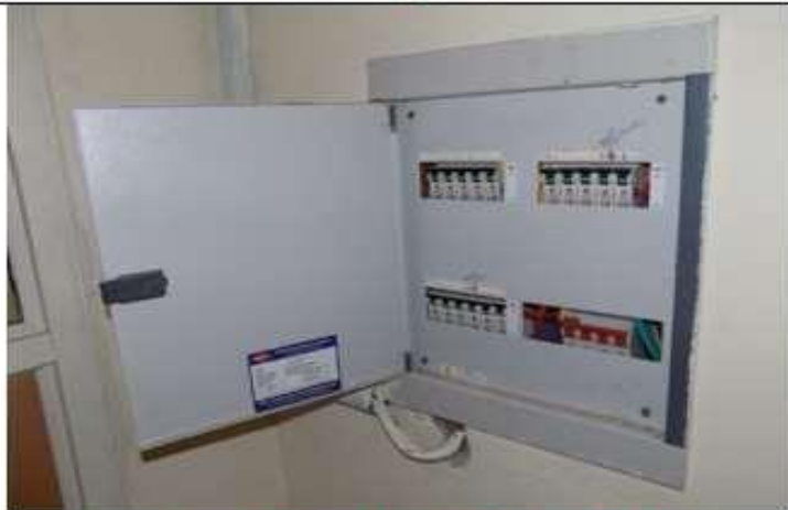
Miniature Circuit Breaker's (MCB's).
