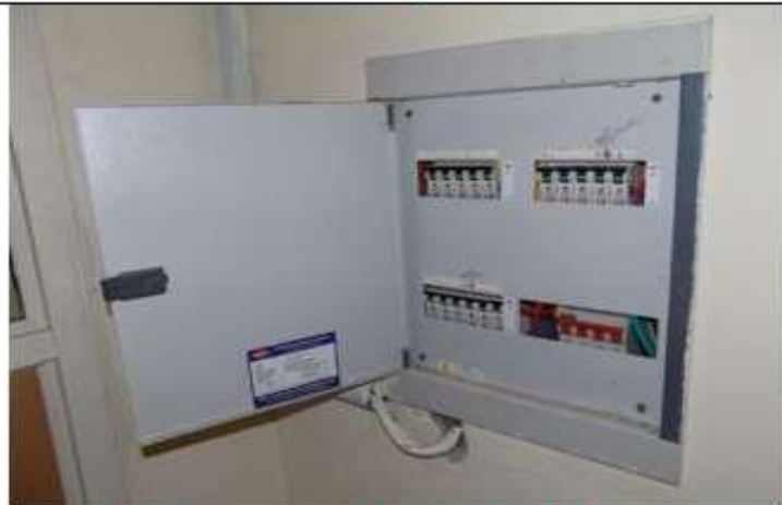
Miniature Circuit Breaker's (MCB's).
